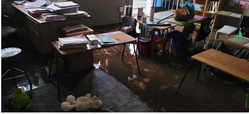
Figure 4- Grade 3 class after water has subsided
